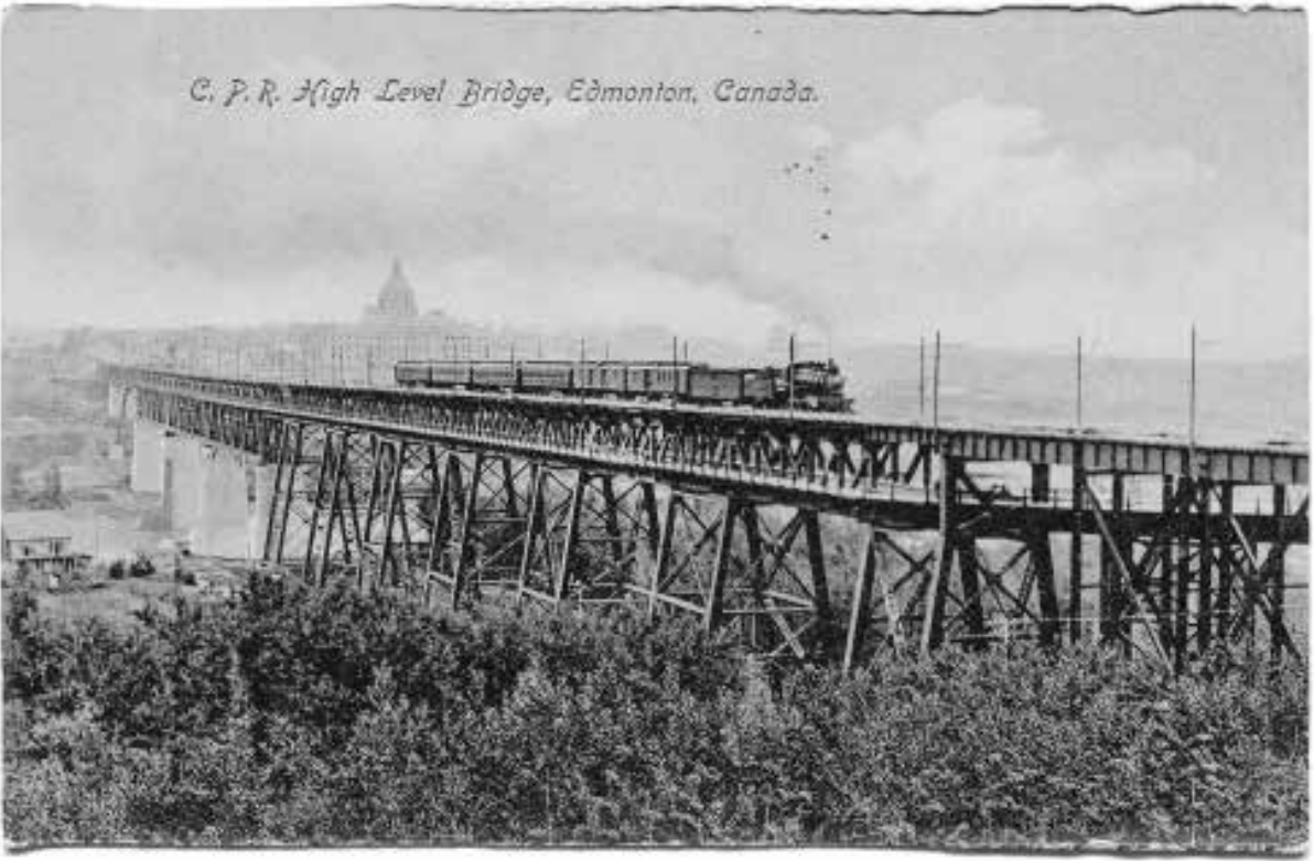
CPR High Level Bridge, Edmonton
